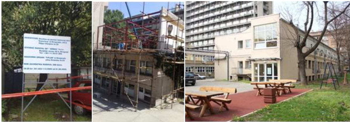
Figure 13. Construction of “The family house”
