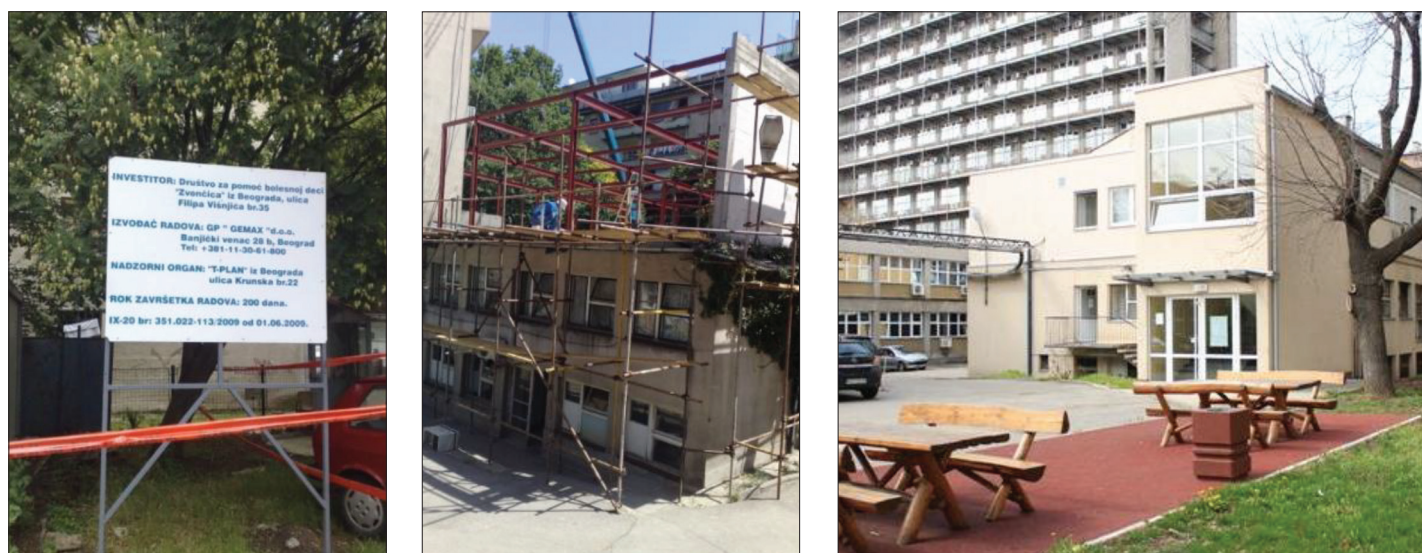
Figure 13. Construction of the Zvončica Parents' House
